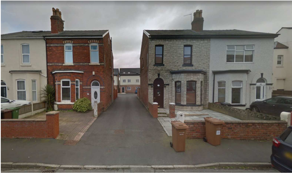
123 Sefton Street - House in the middle with stone façade
