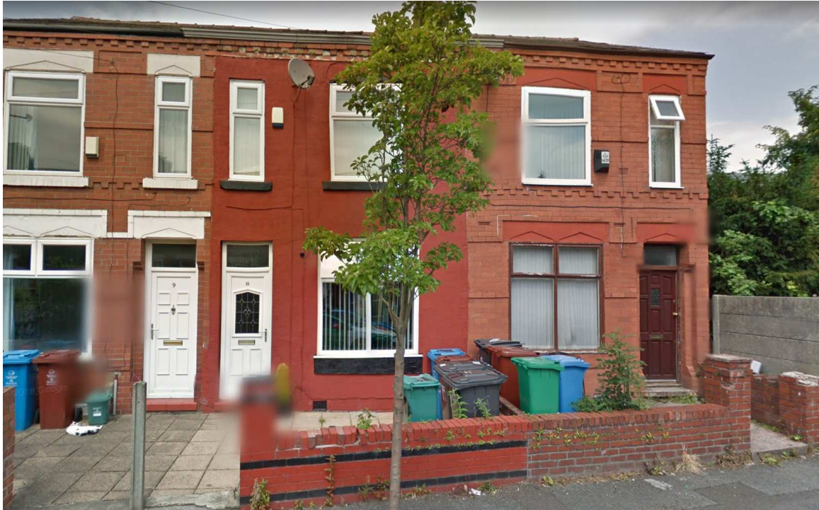
15 Thorncliffe Grove (house on right)
