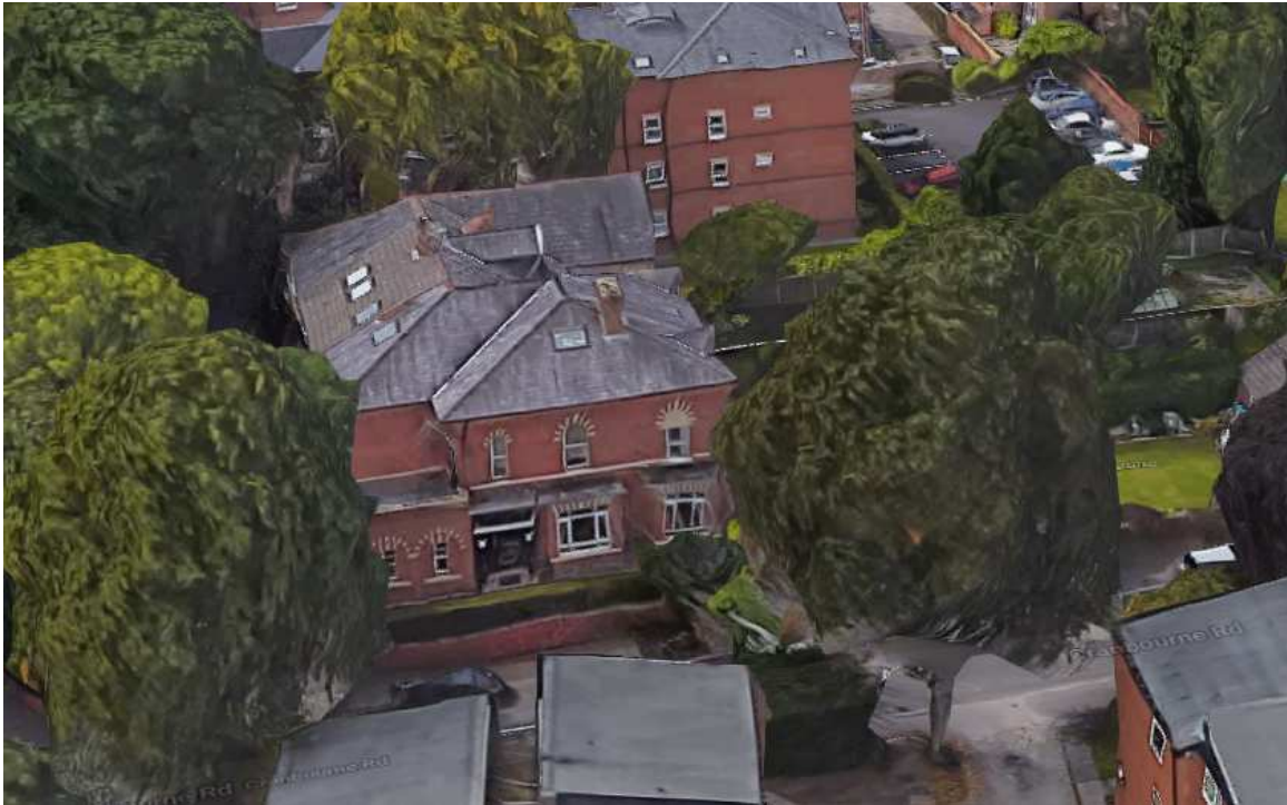
144 Heaton Moor Road (looking at the west side)
