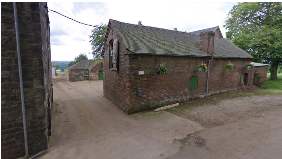
The entrance from Park Lane to the farm yard.
