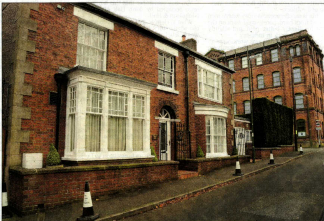
Lyndhurst House, Queen Street. John Hall lived here in the 1870s.
